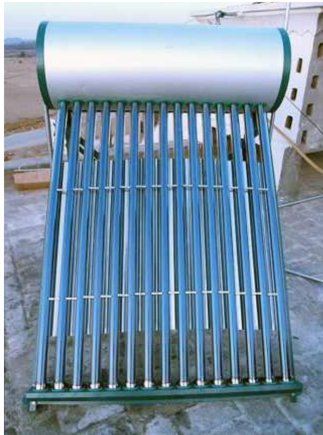
An assembled solar water heater.
